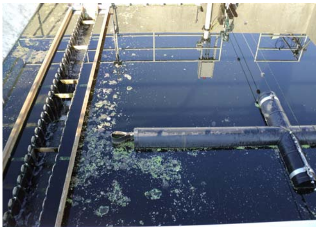
Figure 3.9 Surface skimmer in west clarifier
