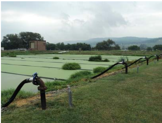
Figure 3.11 Lagoon 2, solids holding lagoon
