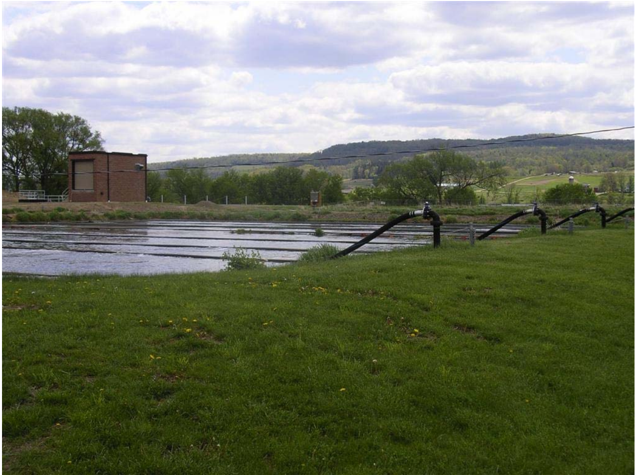
Figure J.3 Solids holding lagoon 2
