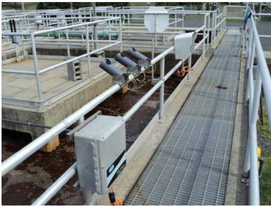
Figure F.3: Stage 2 Air Compressor for NH4Dsc Probe & clamps for probe poles
