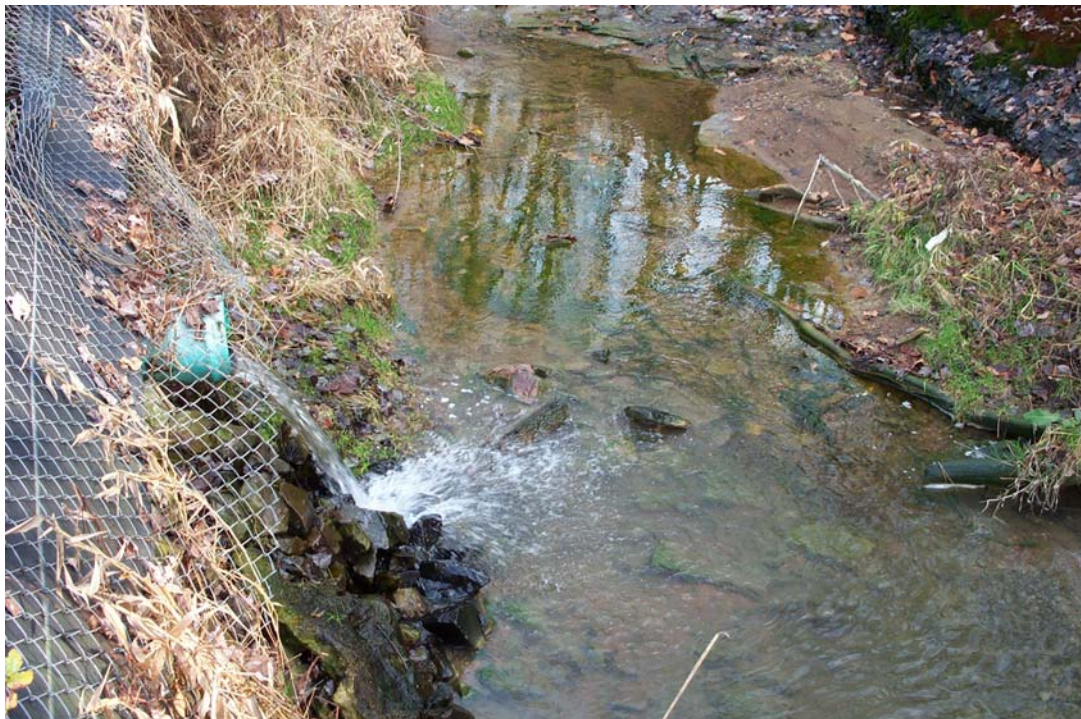
Figure 37. Outfall 001 at Cats Run
