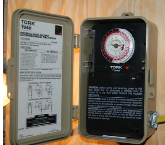
Figure G-10: $40 timer used to control blowers
