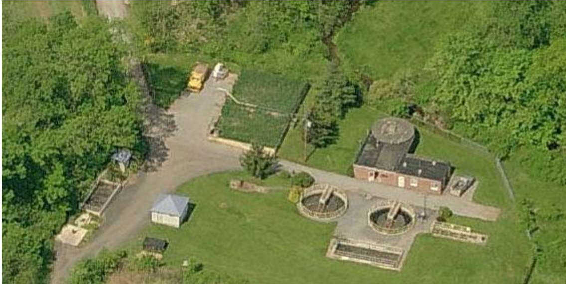
Figure G-1: Treatment System showing three aeration tanks, septic station, control building, and reed beds.
