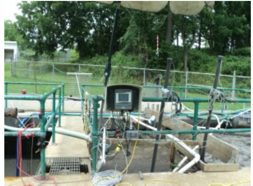
Figure 5-5: Anoxic zone with SC1000 display and 2 probes
