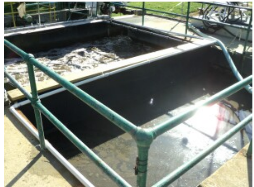
Figure 5-12: Completed wall in place for oxic / anoxic zones
