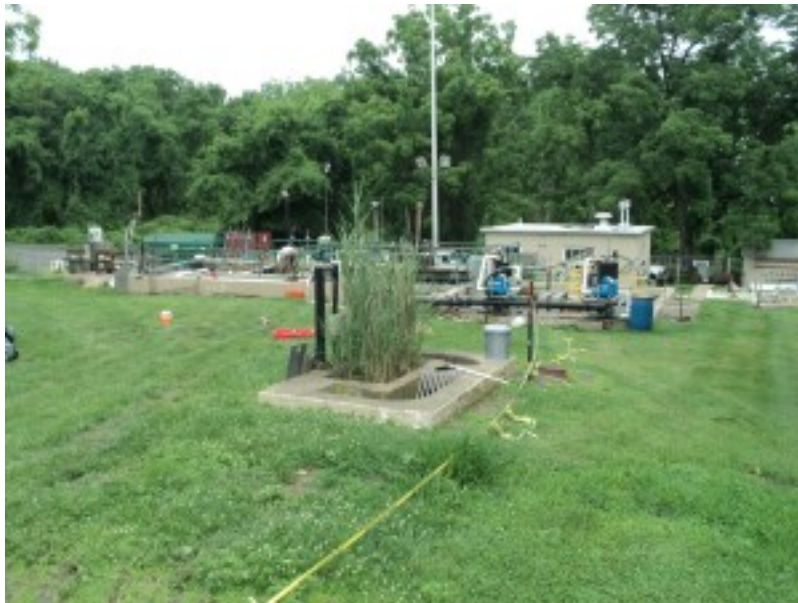
Figure 5-1: Overview of STP from former Comminutor vault
