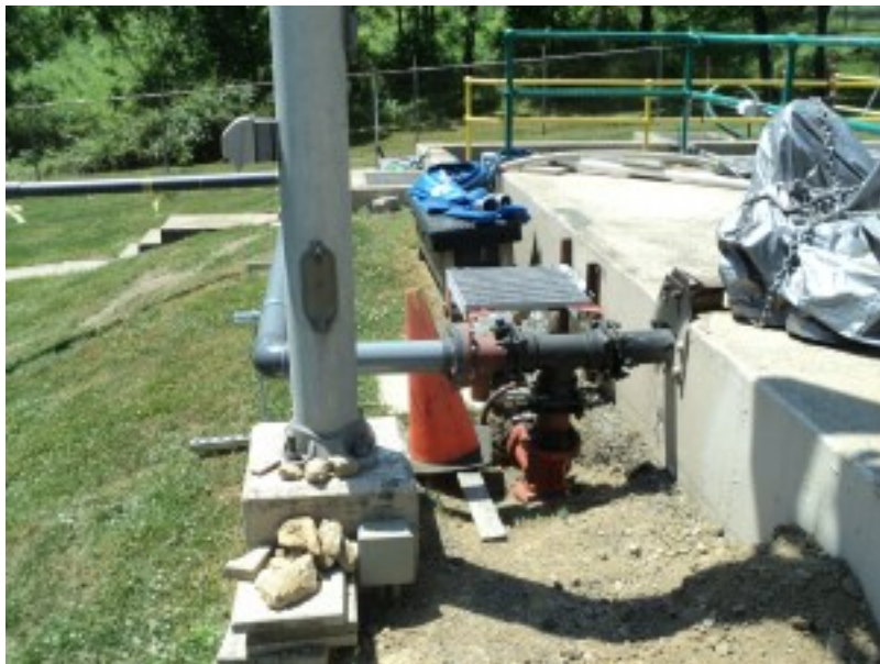
Figure 5-15: Aeration Header Separation in Process
