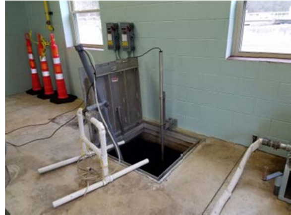
Photo 2: Nutrient probes at Disinfection wet well
