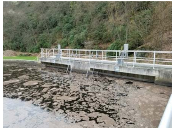
Photo 4: Ditch settling (clarification) stage
