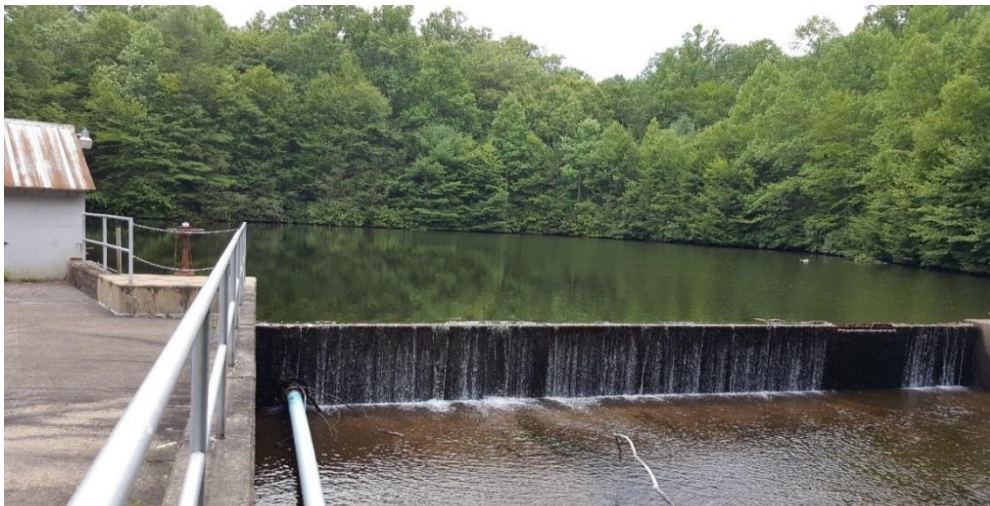
Surface Water Source Retention Basin and Intake Structure
