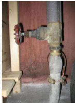
Example of a lead line wipe joint
