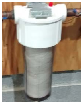
Picture of “wound” style of sediment filter in plastic filter housing
