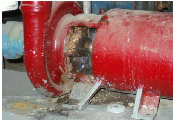
Figure 3.1 Leaking Gland
