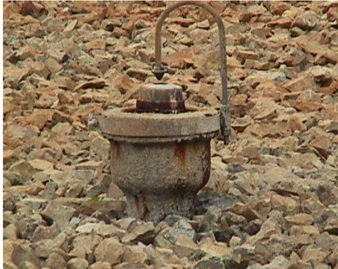
Figure 1.6 Spray Head for a Stationary Trickling Filter
