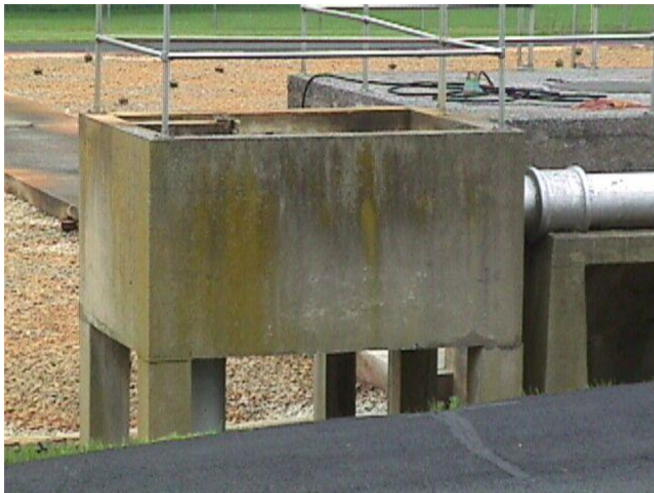
Figure 1.4 Dosing Chamber for Stationary Trickling Filters
