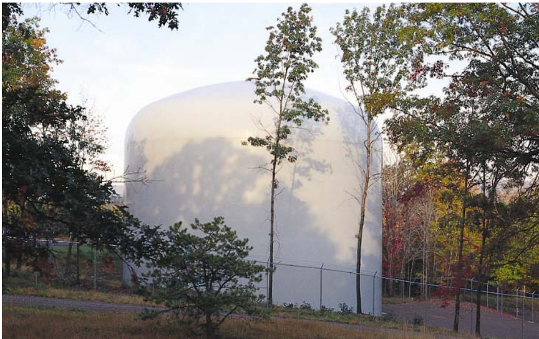
Figure 3.2 – Ground Level Tank
