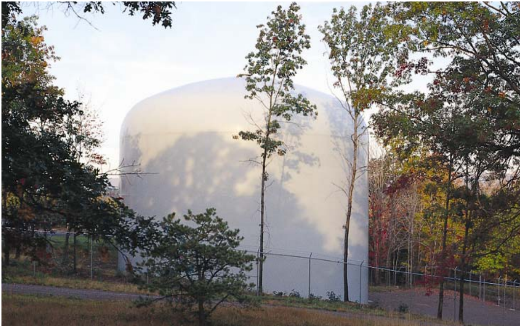
Figure 3.2 – Ground Level Tank
