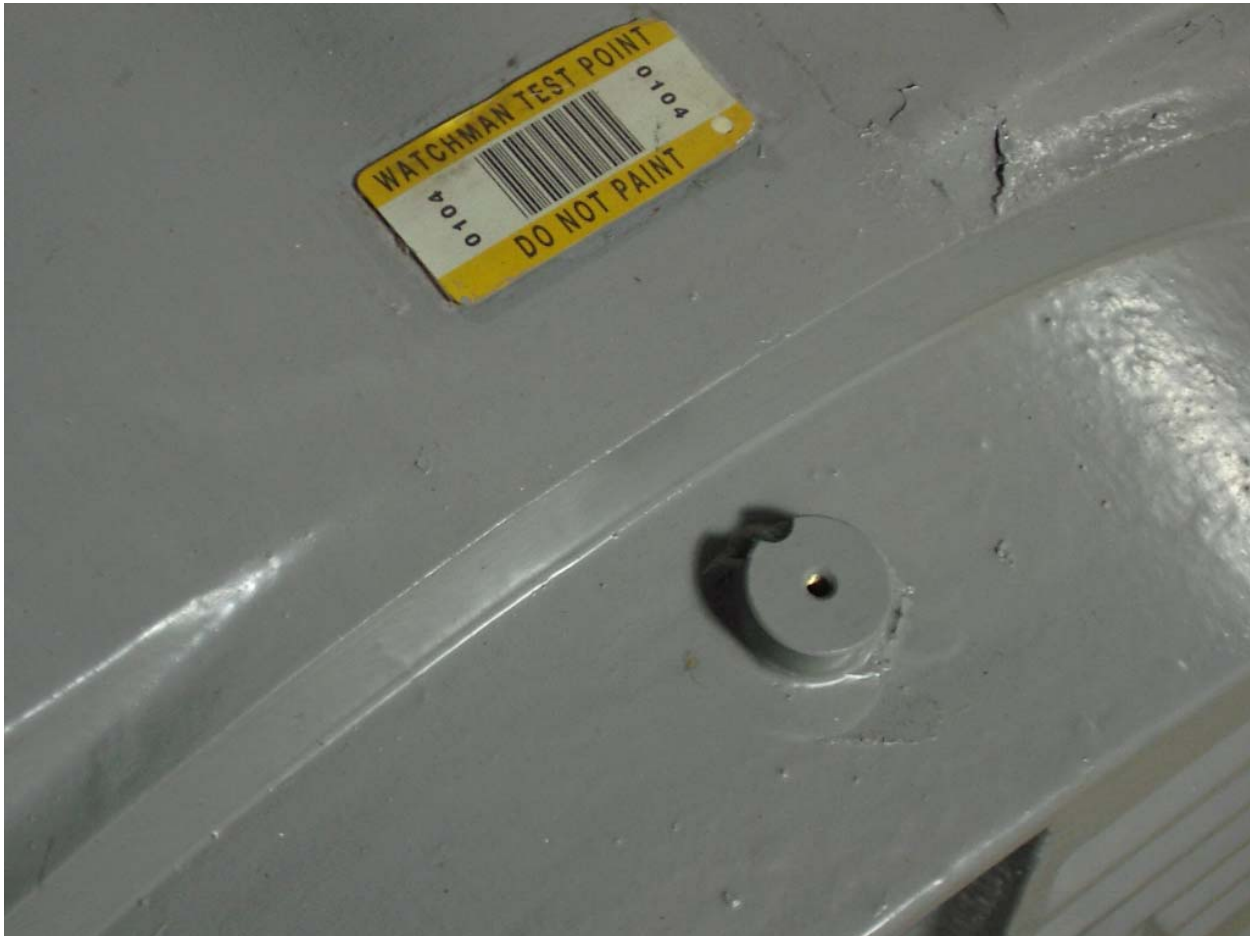
Figure 4.2 Vibration Analysis Point
