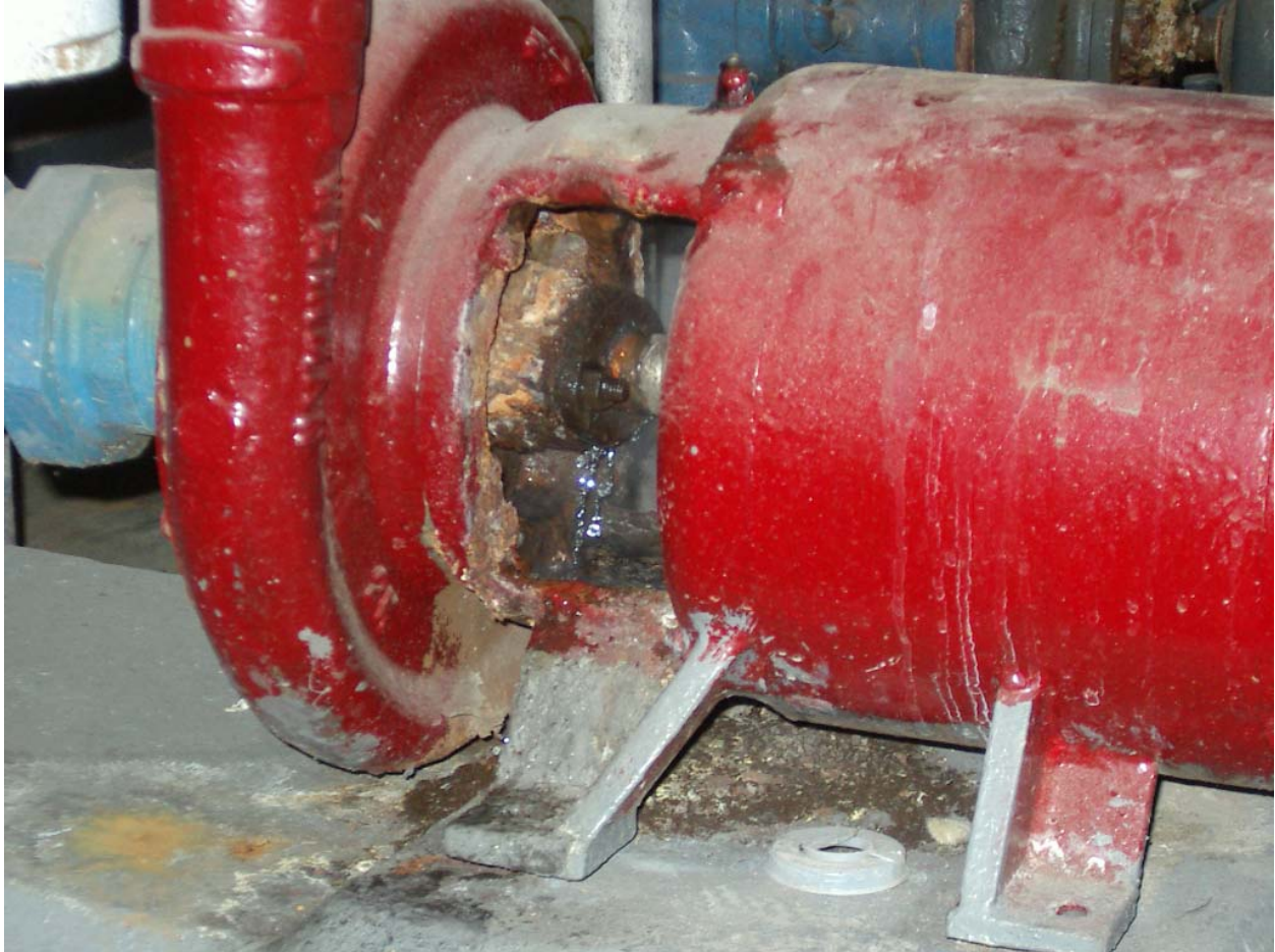
Figure 4.1 Leaking Gland
