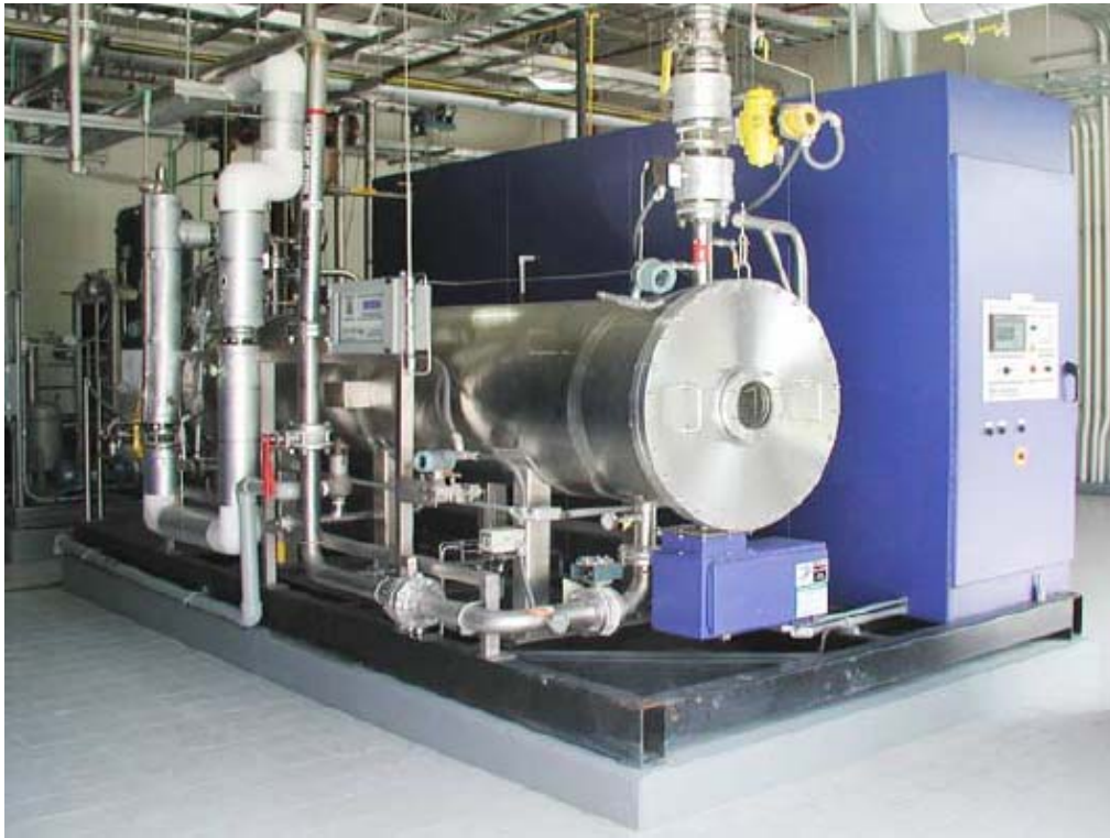
Figure 2.4 – Ozone Generator and Power Supply 2
