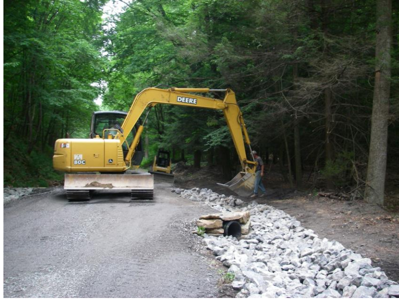
Passive Alkalinity Addition Project on State Game Lands #67 Access Road.
