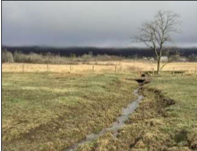
Photo 11: UNT flowing directly into Evitts Creek in need of BMPs.
