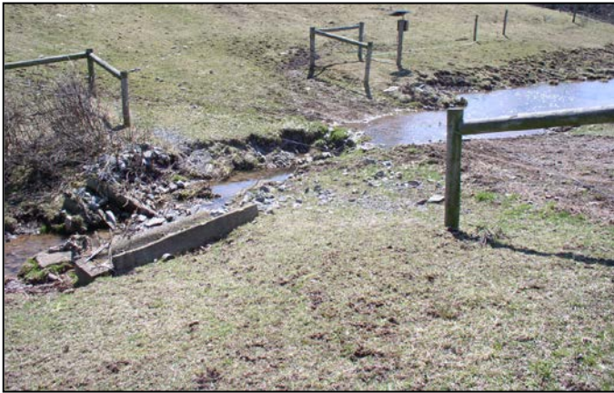
Before installation of a stream crossing and streambank fencing.
