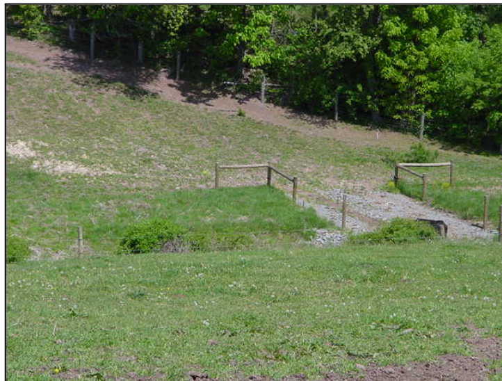
One year after installation of a stream crossing.
