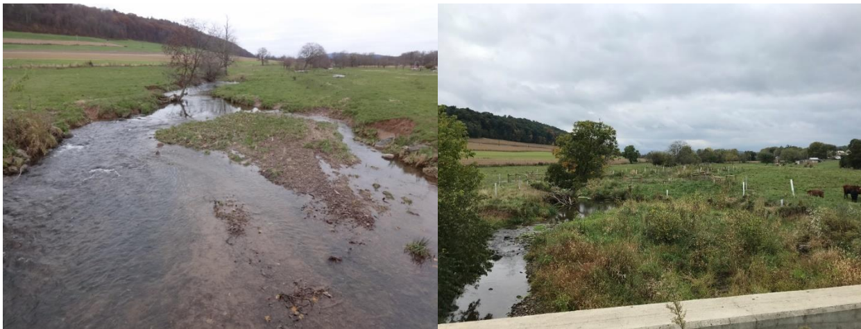
Figure 11: Before (2018) and after (2020) installation of fencing, crossing, and buffer planting at downstream end of Weaver Martin farm, Susqueheca Creek.
