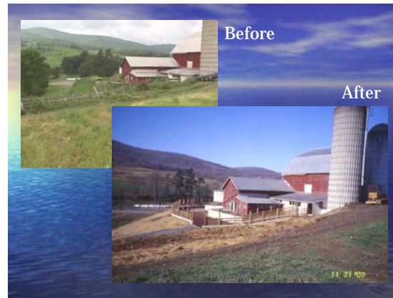
Figure II-02. Barnyard runoff control and animal waste storage improvements.
