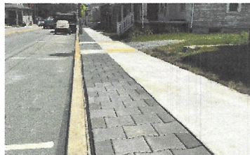
Completed Permeable Sidewalk
