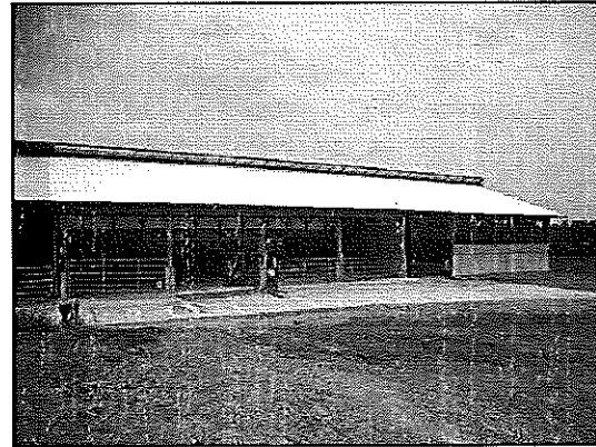
[After] Completion of Animal Heavy Use Area and 60' x 40' x 6' dry stack manure storage. Storage provides 4-6 mo. Capacity
