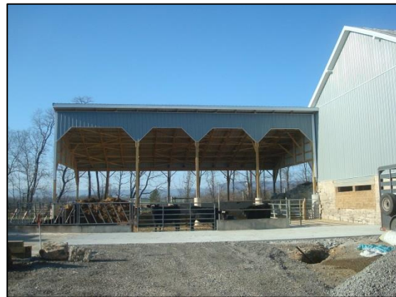
After: Monismith. Roofed heavy use area and waste storage facility.
