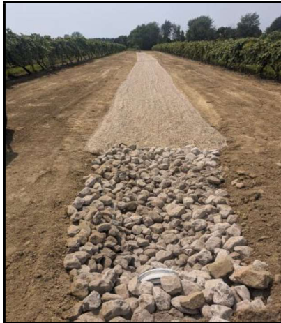
Mid-construction of grassed waterway
