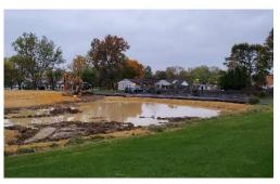
In this series of photos: #1 shows the site prior to any projects – stormwater runoff during rain event with no retention/filtration. #2 shows the same site where the existing swale led directly into the stormwater drain. #3 shows the same site with an improved swale and the wetland basins being constructed
