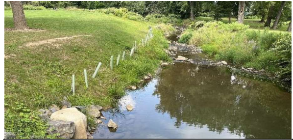
Same section of Arnold's approximately 8 months after single log deflectors were installed and a few months after a buffer was planted.
