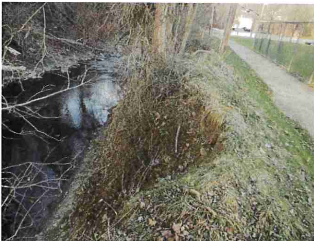
Before: eroding and vertical banks causing sediment to enter the stream.
