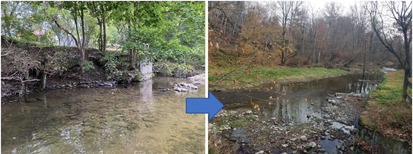
Before photo on left shows the severely eroded and undercut streambanks typical of the project areas along with sediment deposition. After photo on right shows the installed instream habitat structures and newly graded streambanks.
