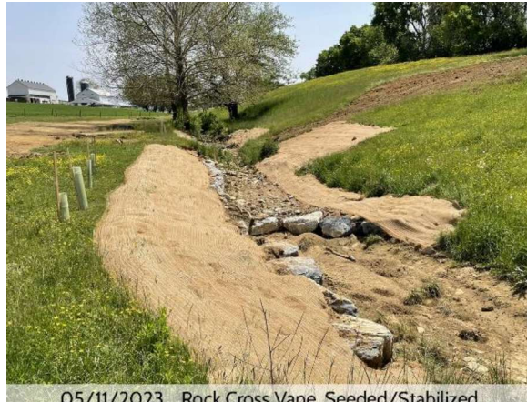
05/11/2023 Rock Cross Vane, Seeded/Stabilized Streambank, and Tree Seedlings
