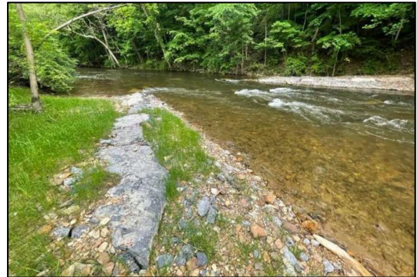
After: Rock cross vanes and random boulder clusters narrow stream channel and provide diversity.
