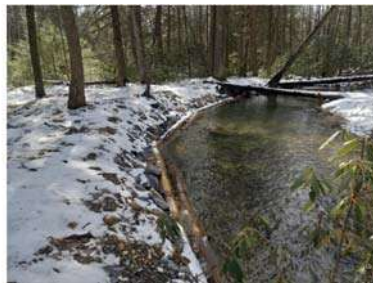
After: Stream stabilized with habitat structure
