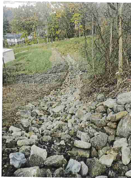
(After) Hillside with installed channel
