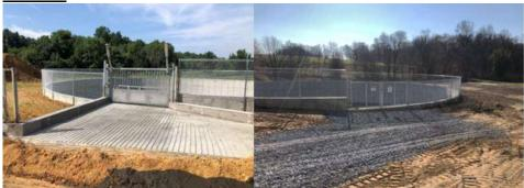
Concrete waste storage facility with safety fencing, gates, manure push-off, and access road to pump-out.
