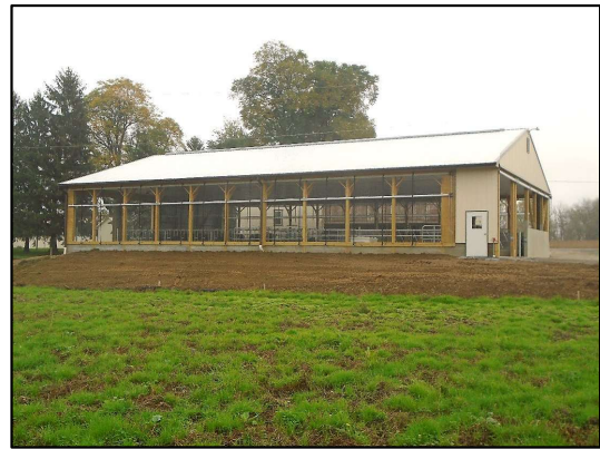
AFTER: New heavy use area and manure storage facility provides a stable location to separate nutrients from stormwater runoff, and prevent sediment runoff into nearby streams.
