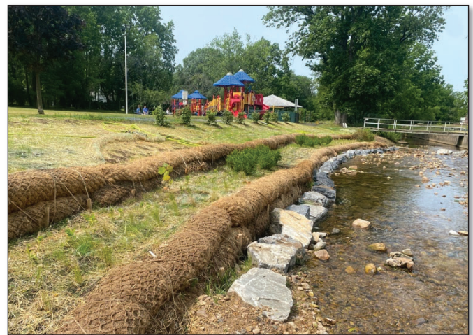
After Streambank Restoration (Regrade, Coirs, Plantings)
