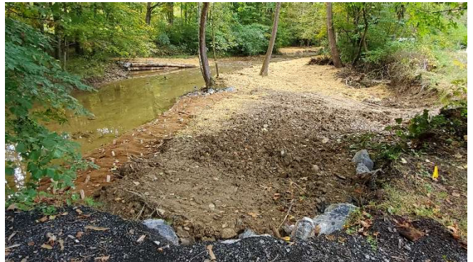
After: The pocket was filled with native material and edged with rock for stability. It was later planted with trees and shrubs. A streamlined, stable stream is the result.
