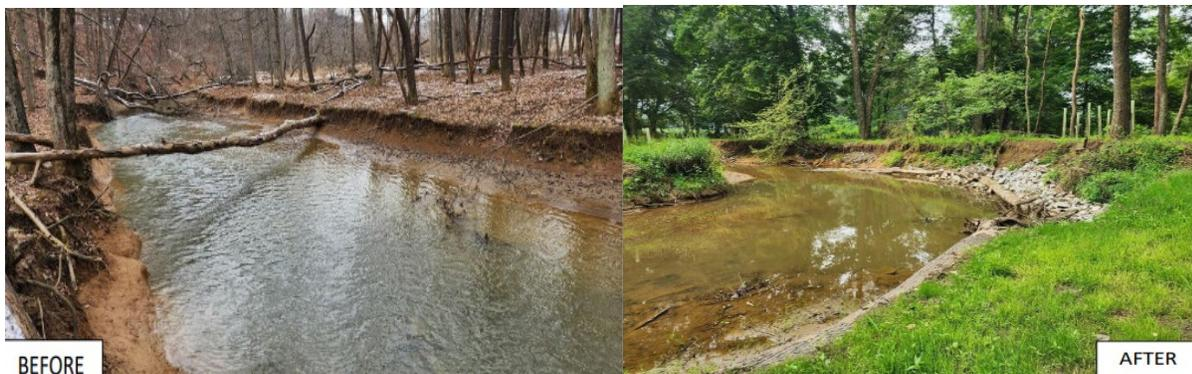
**Project Results** – Five cross vanes with root wads and seven cross vanes were installed. These log vanes deflect water from the streambank and into the center of the channel. This serves to decrease stress on the streambanks as well as creating aquatic habitats in the scour pools that are formed from the redirected flow. With the installation of these cross vanes, 800 linear feet of streambank was stabilized.
