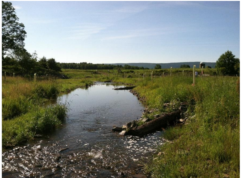
Close up of the multi-log deflectors utilized in the Alba Creek stream corridor rehabilitation project. (2012)
