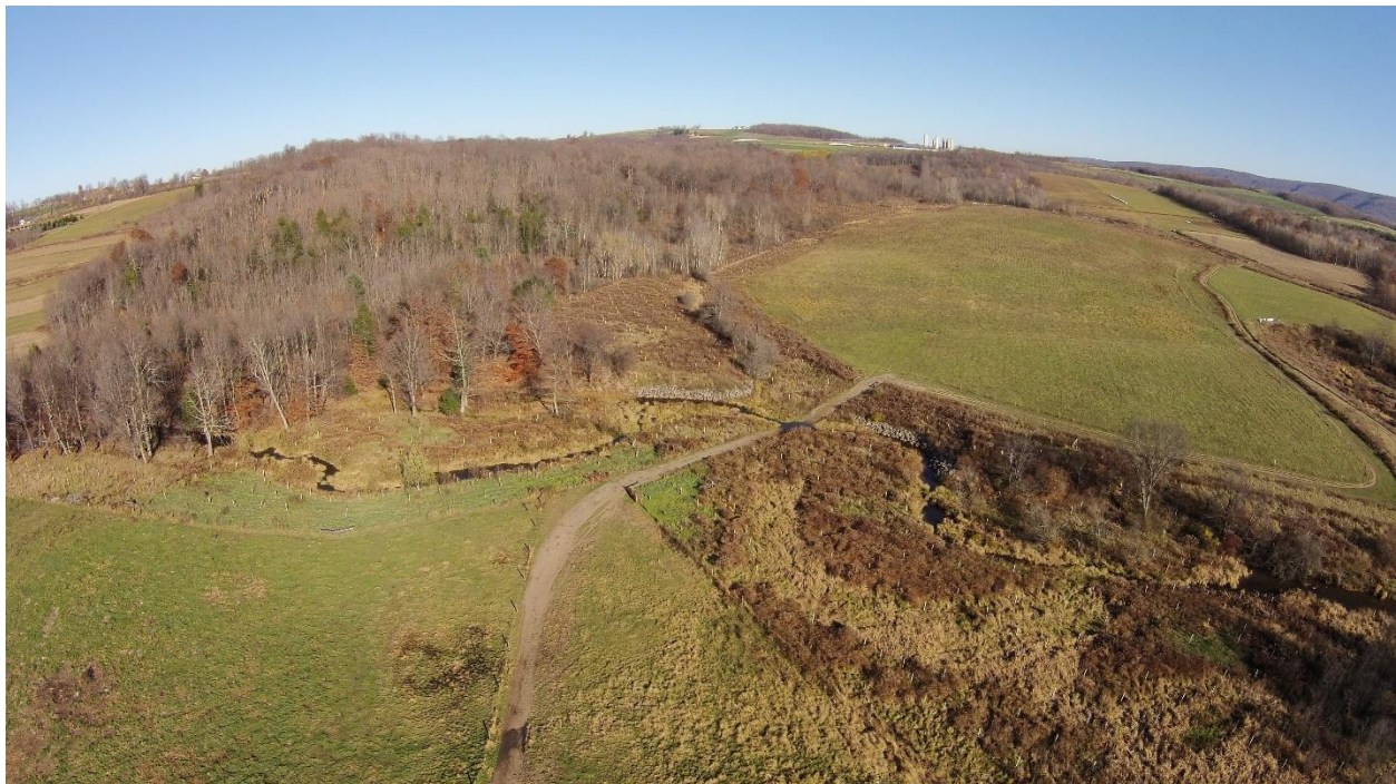
Stream corridor rehabilitation project located within Alba Creek, Bradford County and 1,800' of additional tributaries. Project consisted of riparian buffer, streambank fencing, and streambank rehabilitation. (2012)
