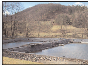
The water treatment plant's sludge beds are shown with Kern Run Dam in the background.
