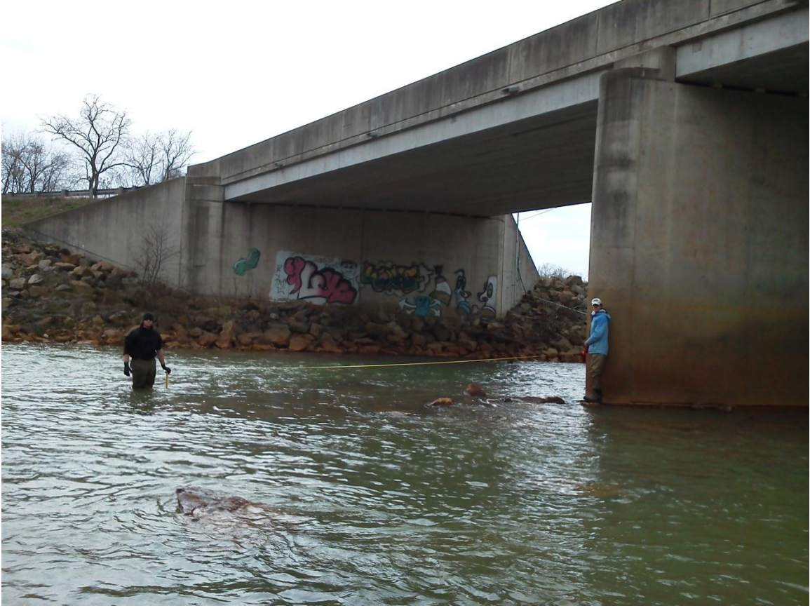
Figure 2. Site location. Picture taken from the bank.
