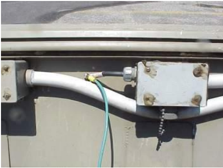
Pic. 1 – grounding to boat hull from generator
