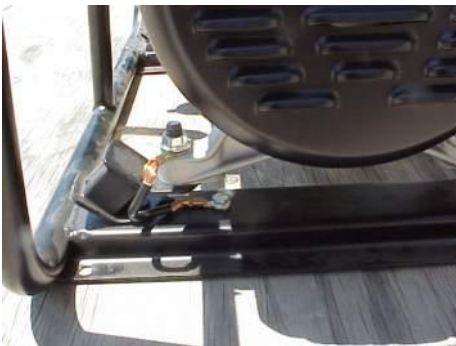
Pic. 3 – grounding generator to generator frame
