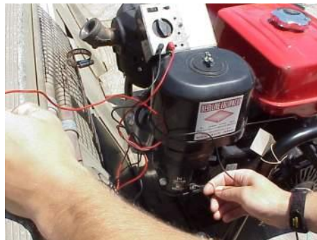
Pic. 4 – checking continuity between generator and Boat hull. (There is continuity)
