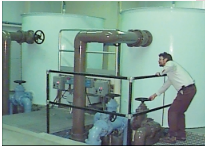
Everett Smeltzer operates a filter flow control valve at the Wrightsville water plant during a filter plant performance evaluation.
