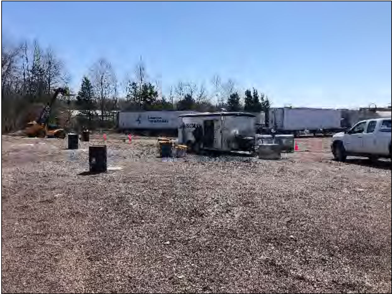
Photo 1: Injection area with RRS injection trailer. Looking South
