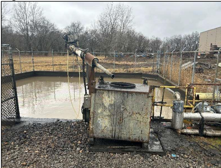
Figure 4. First Flush Tank with oil skimmer
