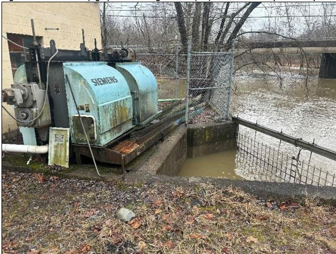
Figure 8. Trash screen (right) and traveling screens (left). DEP's 2025 Inspection Report.
