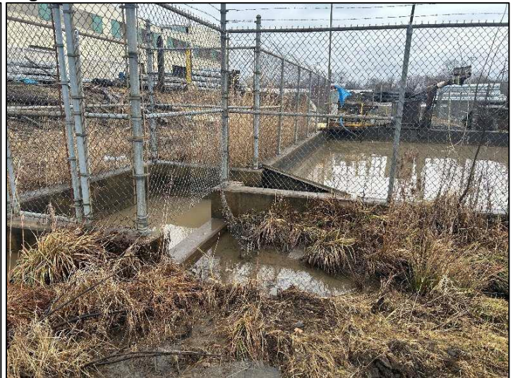
Figure 5. Outfall 006, First Flush Tank weir overflow
