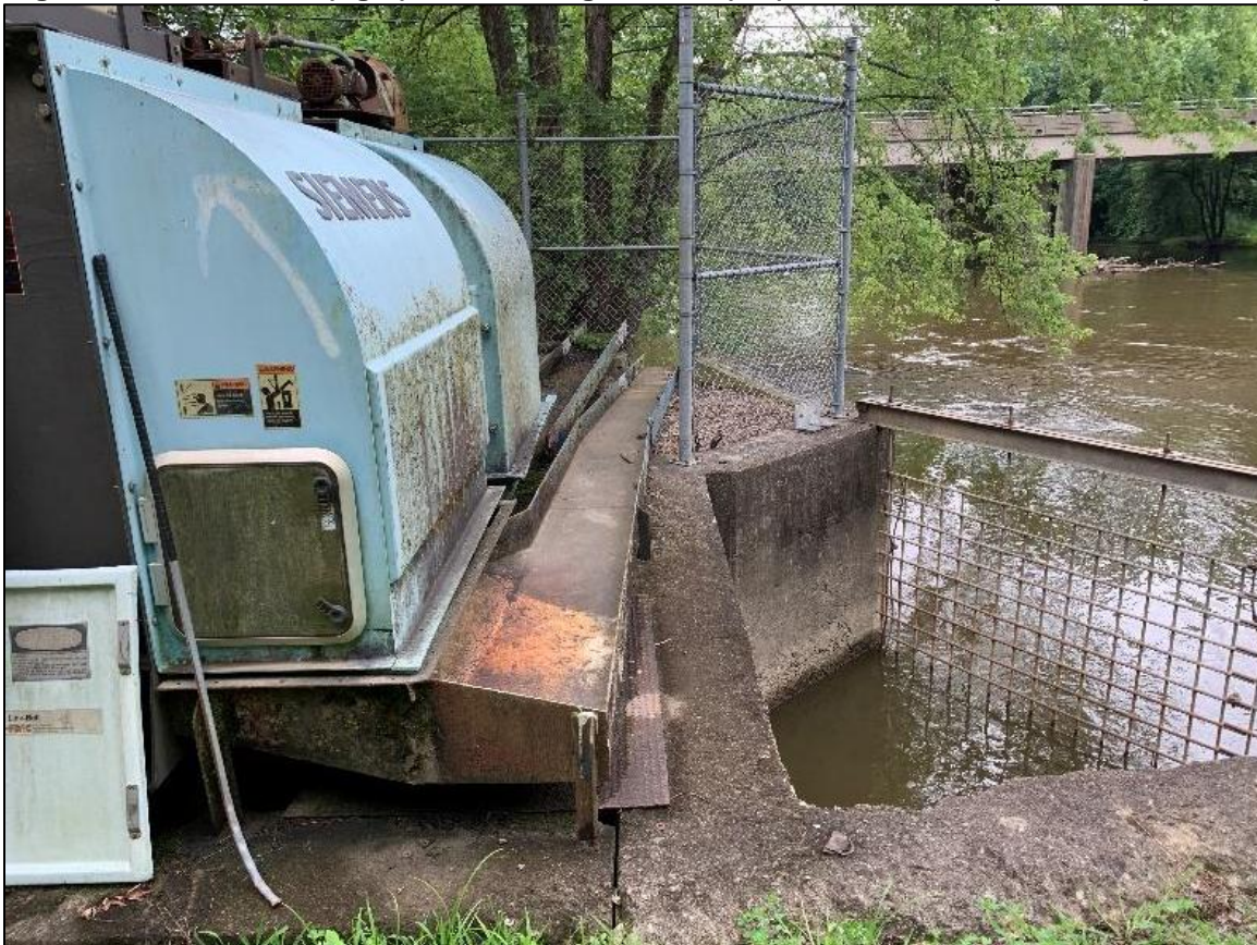
Figure 7. Trash screen (right) and traveling screens (left). DEP 2021 Inspection Report.
