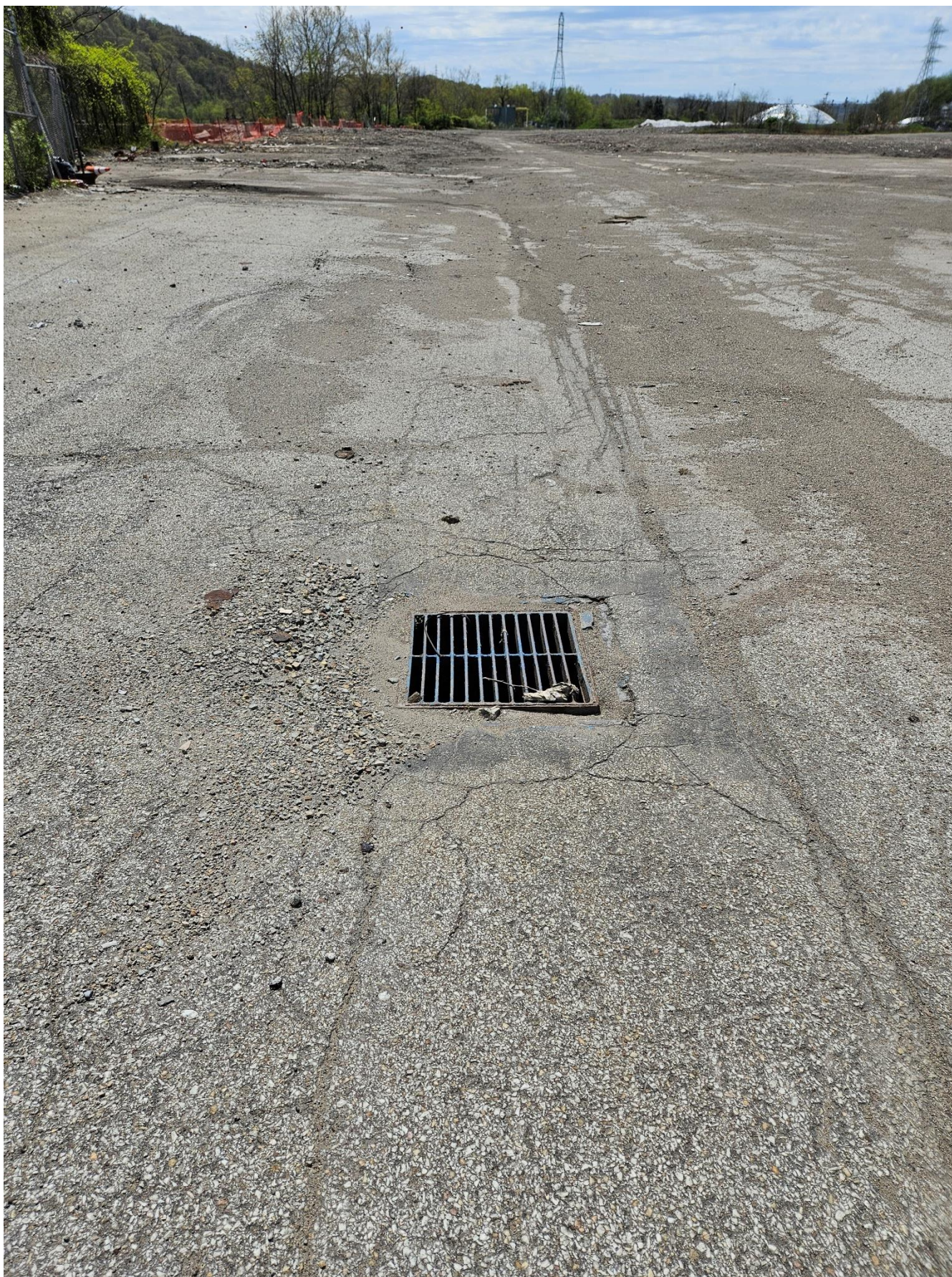
Figure B.5. Outfall 002 representative catch basin
