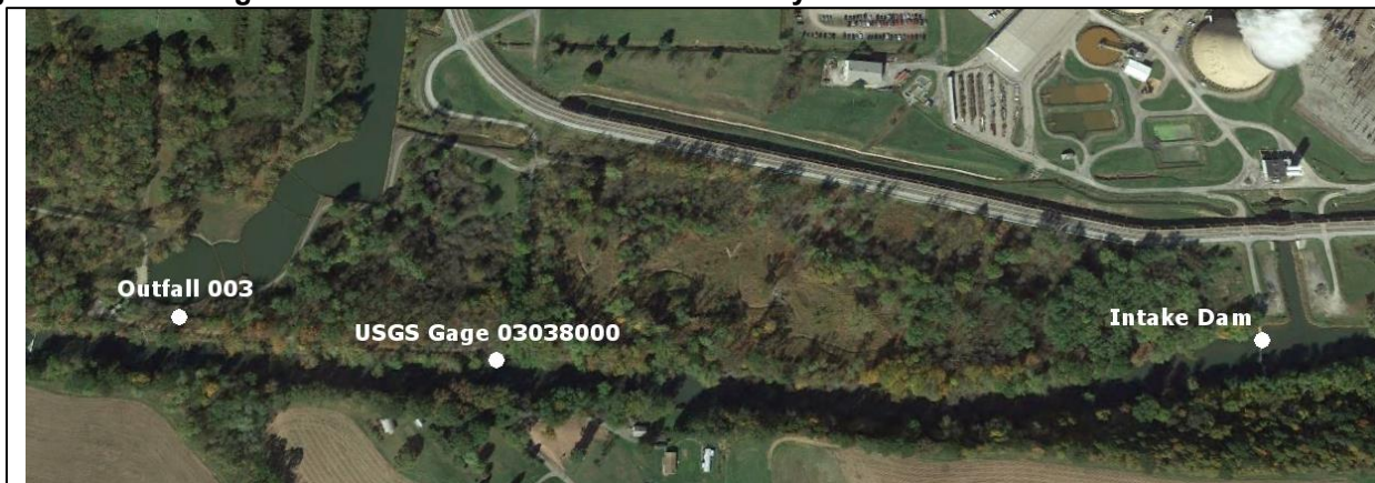
Figure 1. Aerial Image of Crooked Creek Downstream of Keystone's Intake Dam
