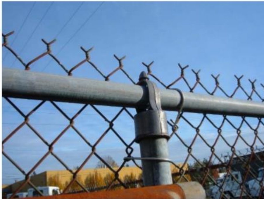
Galvanized chain-link fence can be a major source of zinc, especially when the fence is on paved rather than vegetated ground.
