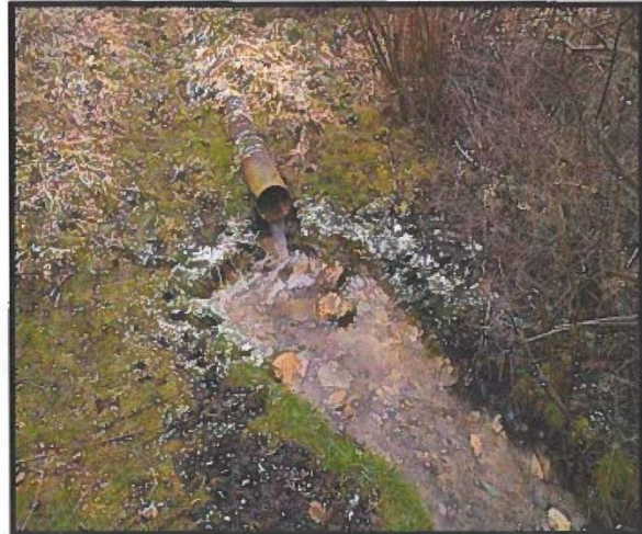
Figure 3. BWWTP treated effluent outfall pipe.
