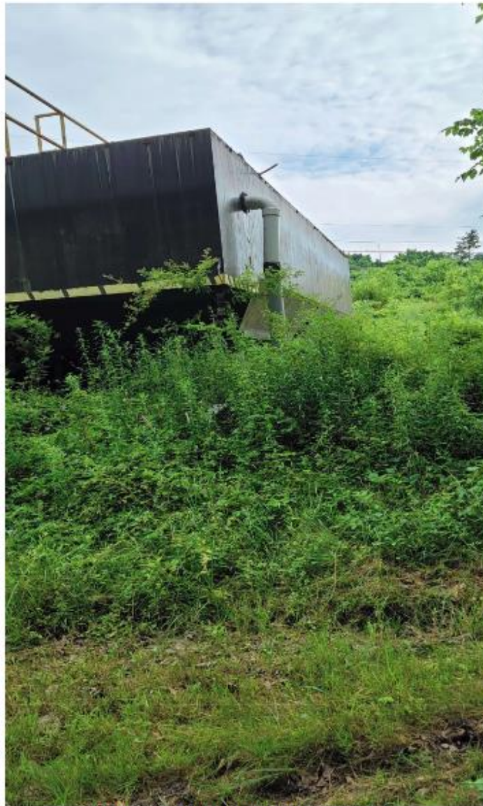
Figure 4. Picture showing abandoned STP.
